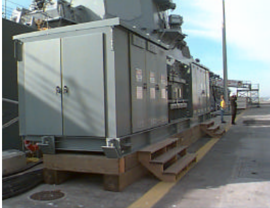
Figure 12-2 A skid-mounted substation
