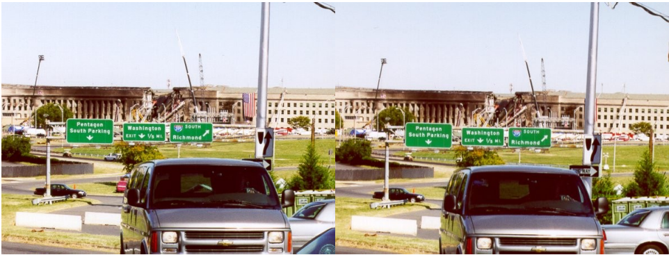
Pentagon Damage from terrorist plane crash on September 11, 2001 as seen from the Navy Annex Photographs taken Saturday, September 15, 2001 By Norbert Doerry
